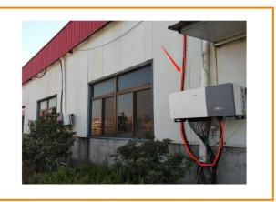
**Suggestion:** Remove part of the external bushing at the wire entry hole of the wiring compartment and prohibit the bushing from directly entering the inside of the inverter. This will prevent rainwater from flowing into the inside of the inverter.
