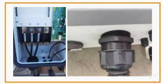
**Suggestion:** Check whether the cable entry hole is well plugged and whether there is a missing PG head. In low level installations, rainwater may splash into the inverter when it rains, or the inverter may be soaked in water. There may also be condensation problems in humid environments. Ensure the cable entry hold is well plugged and will not let water in.
