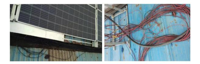
③Poor grounding: Good grounding has two functions. The first is to effectively release the capacitive leakage current of the system to avoid excessive accumulation; the second is to ensure the safety of the system. If the grounding is sufficient and a leakage incident occurs, the leakage current will be sent to earth and will not cause an electric shock.
