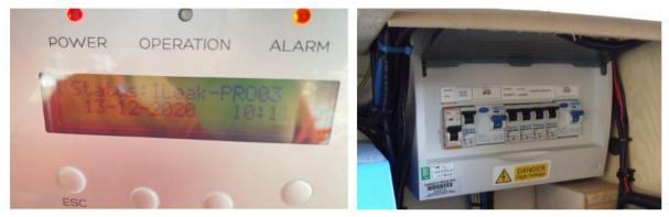
**Likely Reason:** This fault indicates that the inverter and the leakage current protector have detected leakage current from the PV system to the ground.
